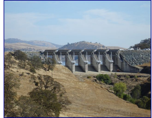
MID's Gated Spillway
