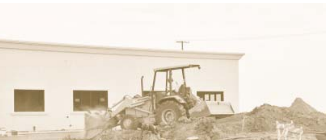
CREATIVE PLUMBING NEARS COMPLETION.
