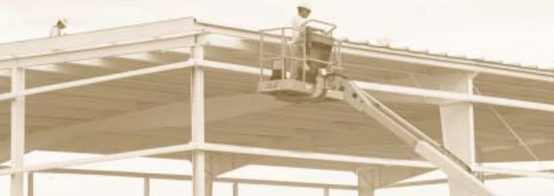
CLENDENIN CONSTRUCTION WAREHOUSE.
