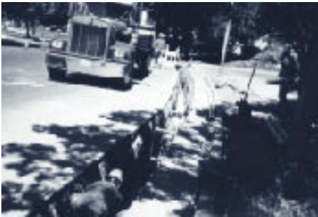
Installing underground electric lines.
